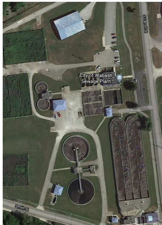
Figure 4-6: City of Wabash Sewage Plant
